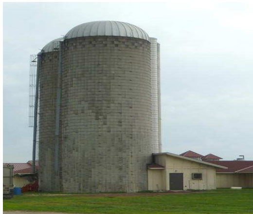
Figure 5. Concrete stave tower silos.
