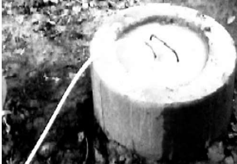
Fig. 1.3: Sub-Surface Concrete Bio-digester (Source: Tajudeen, 2011)
