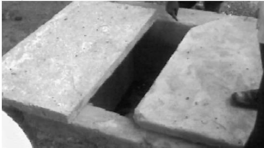
Fig. 1.3: Sub-Surface Concrete Bio-digester (Source: Tajudeen, 2011)
