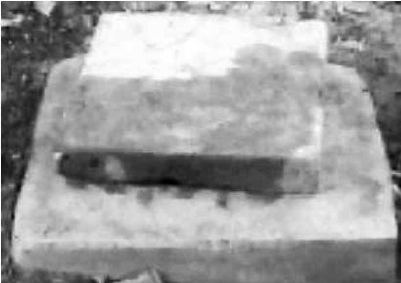
Fig. 1.2: Underground Chinese Batch Type / Indian Dome: Feed Chamber (Source: Tajudeen, 2011)
