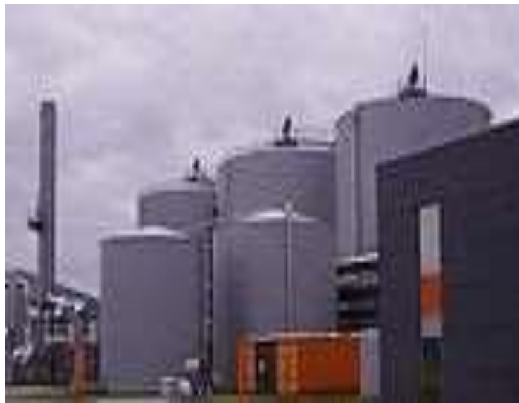
Fig. 5.9: Anaerobic Digestion Component of Lübeck
