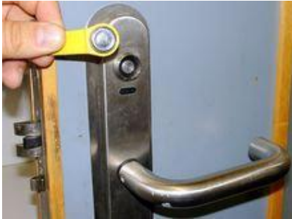
Fig .4.2: An Electronic Access Control
