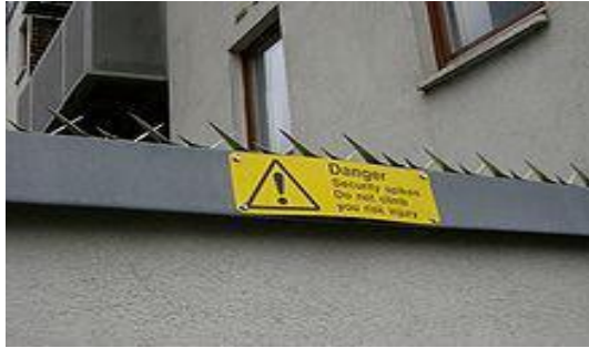
Fig. 4.1: Spikes atop a Barrier Wall
