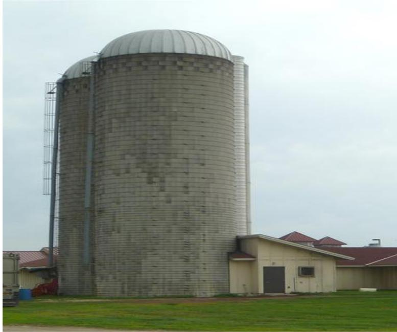
*Figure 5. Concrete stave tower silos.*
