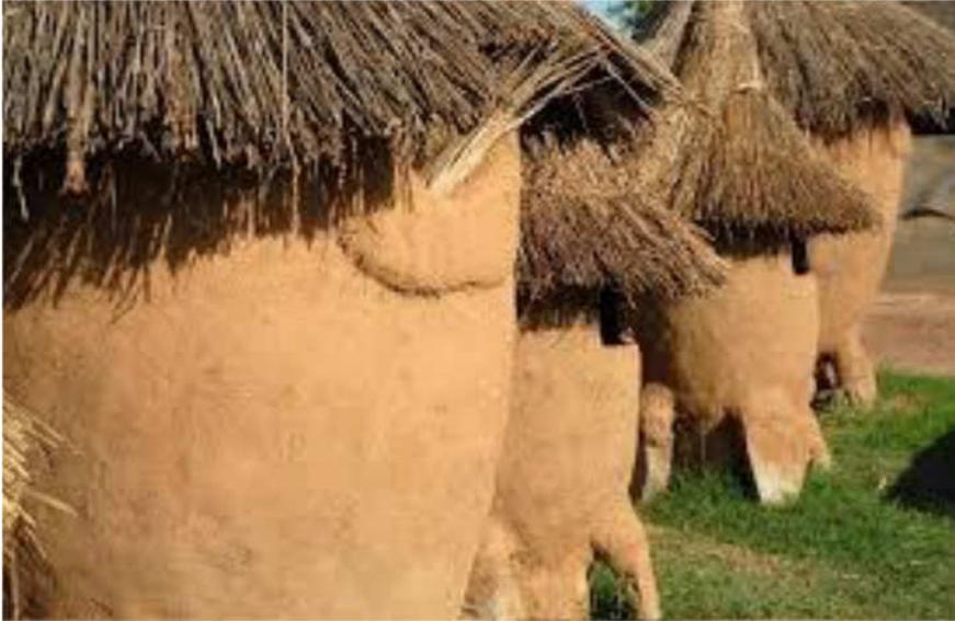
Fig. 7: Mud silos (“Rhombus”)
