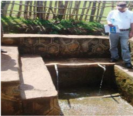
Figure 2: A protected spring (Photo: WaterAid, Ethiopia)
