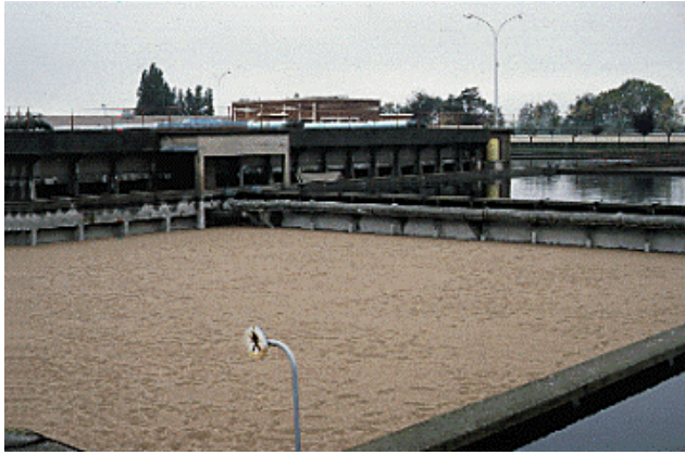
Fig. 11: Slow Sand Filtration Drained slow sand filter in foreground Operating slow sand filter in background
